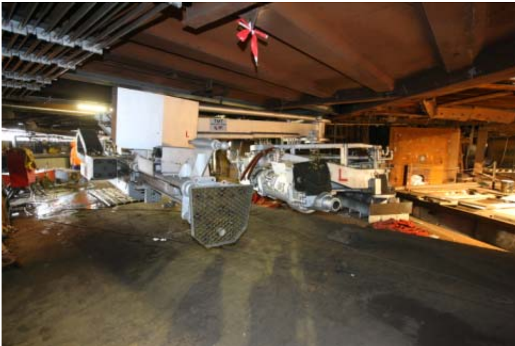
Figure 8. Cast house machines.
