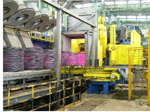
Fig. 9. Coil directly charged onto walking beam conveyor
