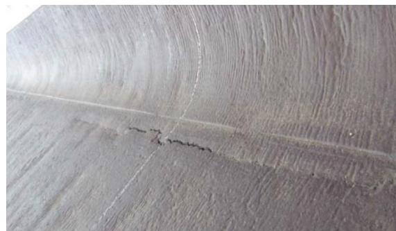
Figure 10. 1050 mm wide beam blank. Longitudinal crack between web and fillet [11].
