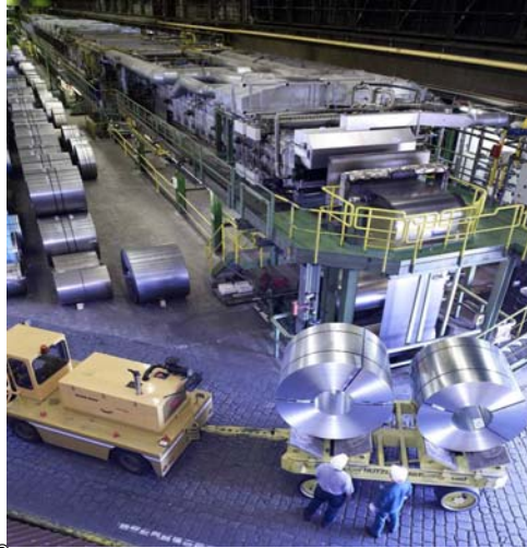
Figure 4. In 2006 the REBOX ® DFI unit was installed at the entry side of the galvanising line at TKS' Fintentrop Works, where it has resulted in 30% increased production capacity and elimination of the use of a pre-cleaning section.
