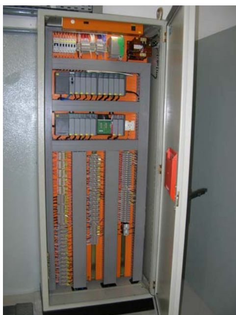
Figura 6 Painel com PLC
