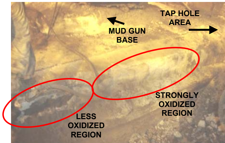
Figure 3. Strong oxidation region caused mainly by water steam
