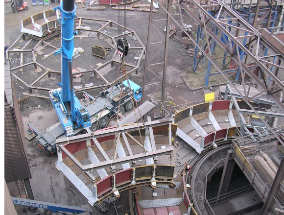
Figure 6: Installation of an extended sinter cooler
