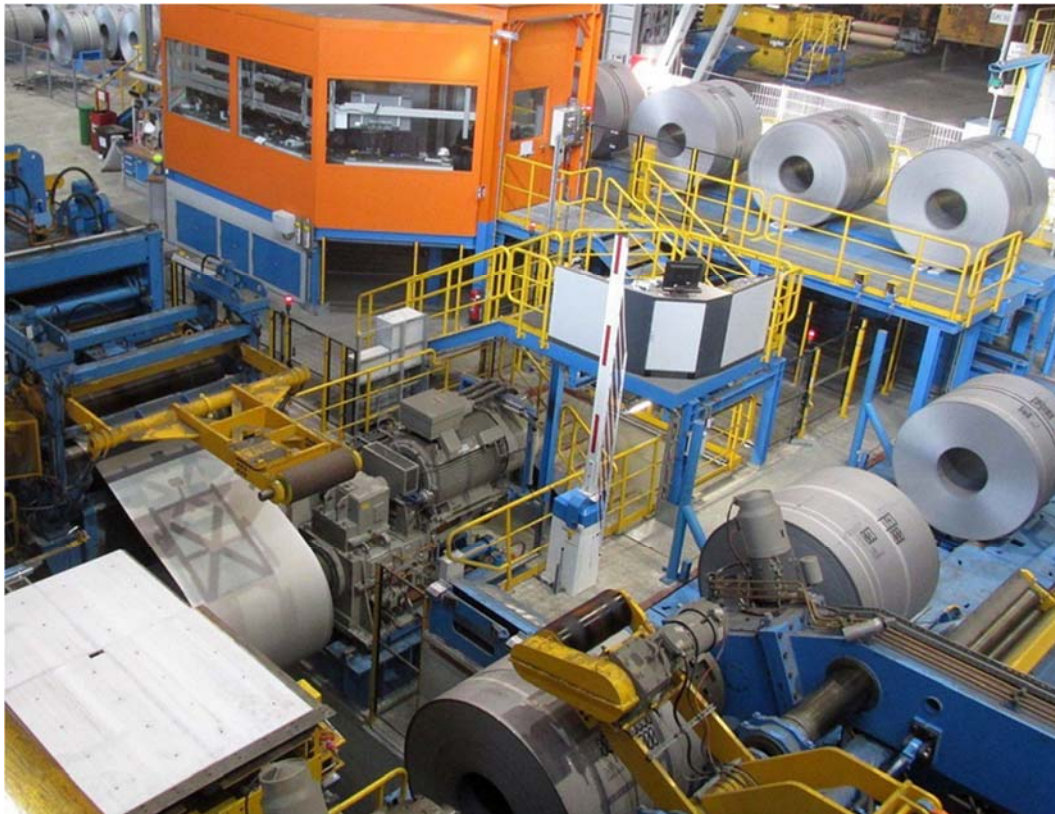
Figure 8. New entry area equipment with walking beams, coil car, auxiliary uncoiler and pay-off reel.
