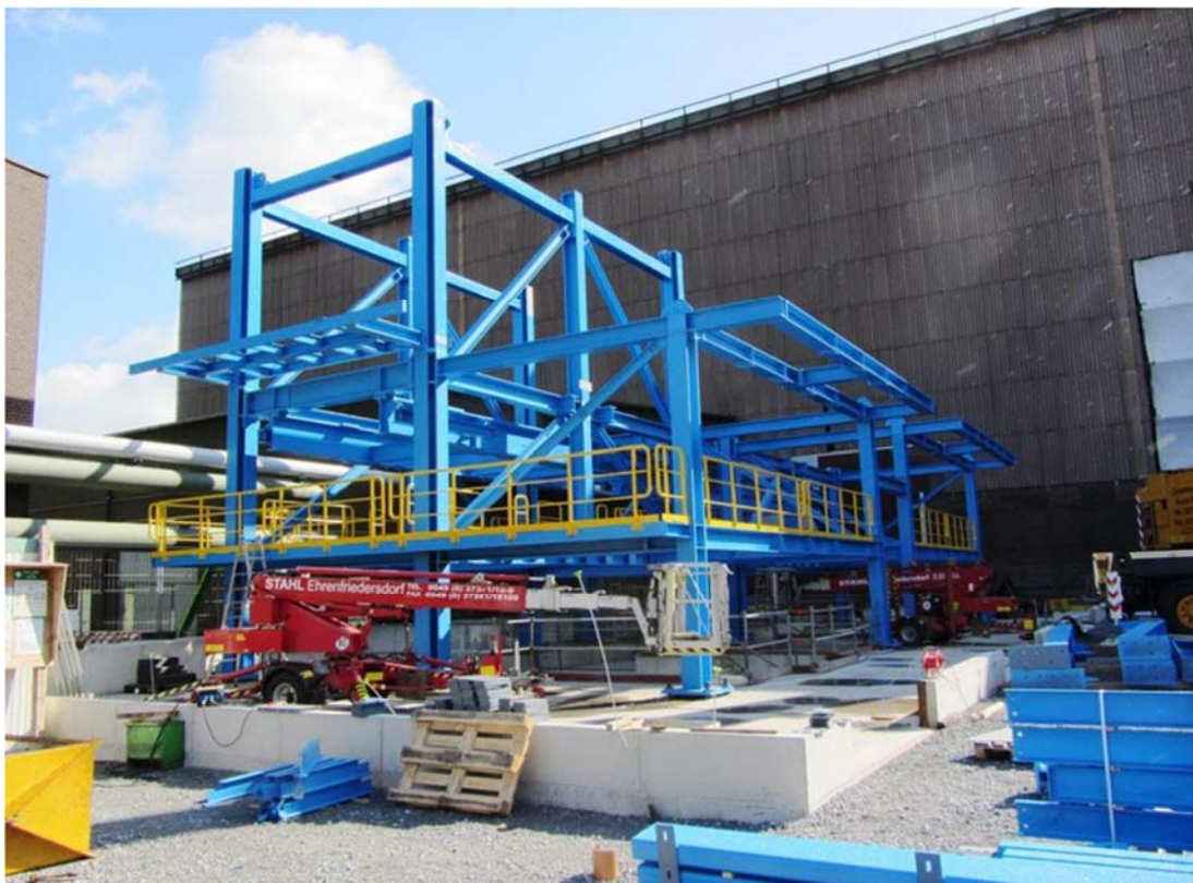
Figure 6. Start of structural steelwork looper towers.
