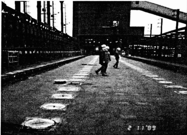
Fig. 5 Oven Roof after Rehabilitation
