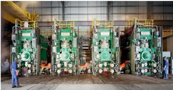
Figure 1: 4-stand CSP ® finishing mill train at Nucor Crawfordsville in 1989
