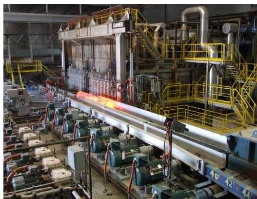
Fig. 4: Walking beam type Re-Heating Furnace.
