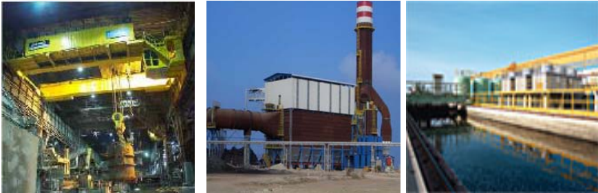
Figure 18. Danieli Cranes, FTP and WTP.
