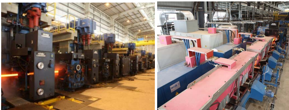
Figure 17. Danieli rolling mill and induction heater.
