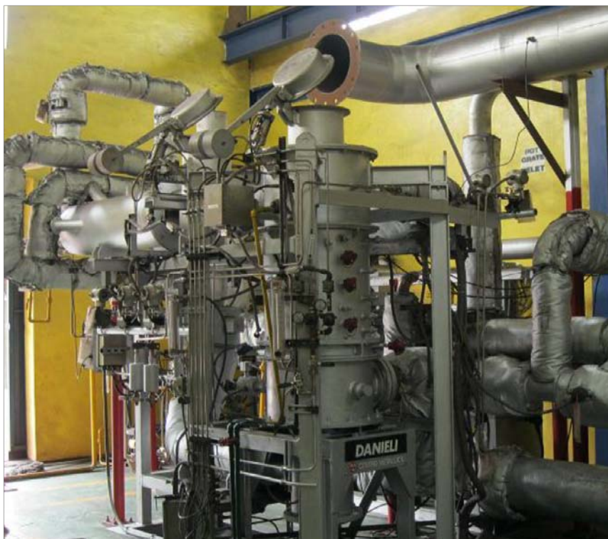
Figure 4 - AHMSA Pot Grate Installation
