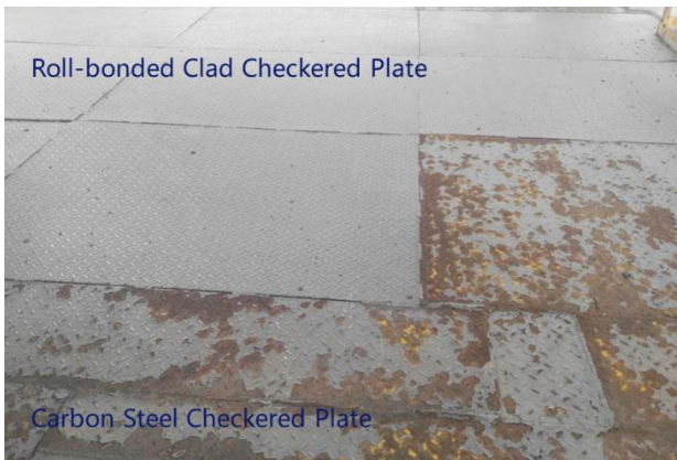
Figure 12. Comparison of two kind of checkered plates after two years of use
