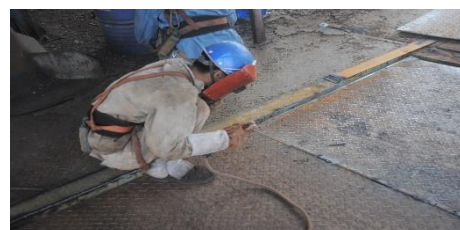
Figure 11. The construction of roll-bonded clad checkered plates
