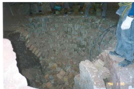
b) Remaining checker bricks.
