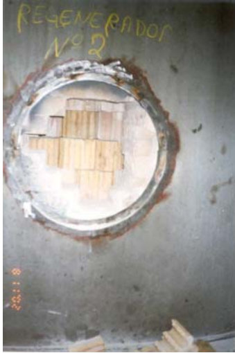
b) Laying Fresh Bricks and Checker Bricks Rebuilding lining.
