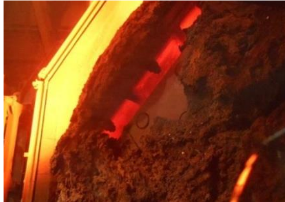
Figure 7. Hot Spot in the Mouth Area Due to Post-Combustion. Source: voestalpine
