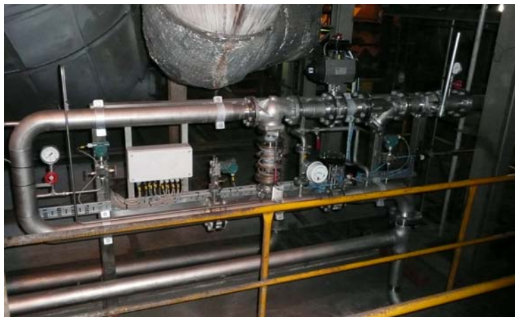
Figure 7: Compact oxygen flow train installed on the walking beam furnace at SSAB - Borlänge in Sweden.
