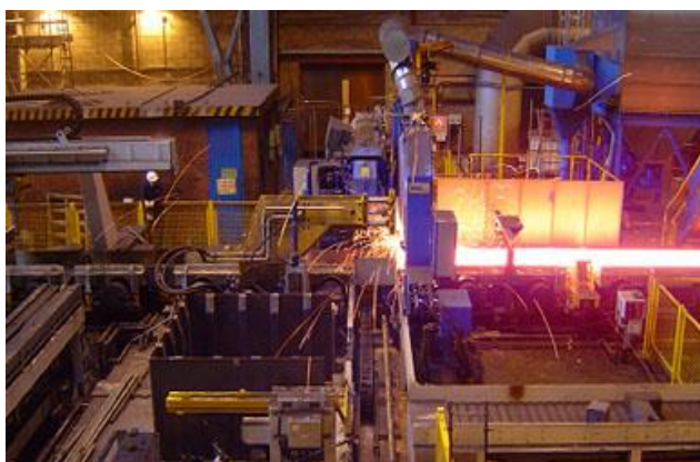
Figure 7. BRAUN abrasive cut-off machine, type TS 16 W (for 1600 mm cutting wheel diameter), for hot cutting of blooms in primary mill (TATA Engineering Steels, Rotherham, UK).
