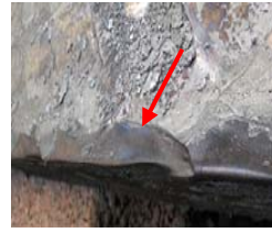
Example of poor edge scarfing technique that can result in plate edge defects, corner too sharp
