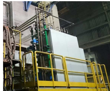
Figure 5: Control cabinet outside the dog-house
