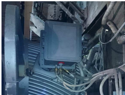
Figure 4: Receiver unit mounted outside the water cooled duct.
