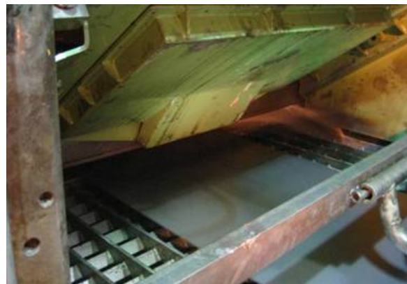
Figure 12. T-Clean: blower type Dry Strip system by SMS Siemag with extended fume suppression and low noise level.
