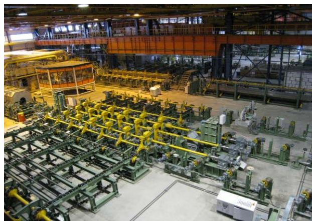
Figure 4: Quenching tank area overview.
