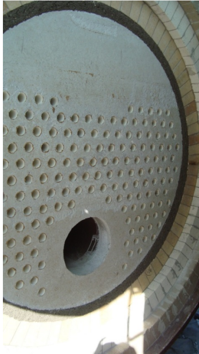
Figure 12. New lining of the waste heat boiler.
