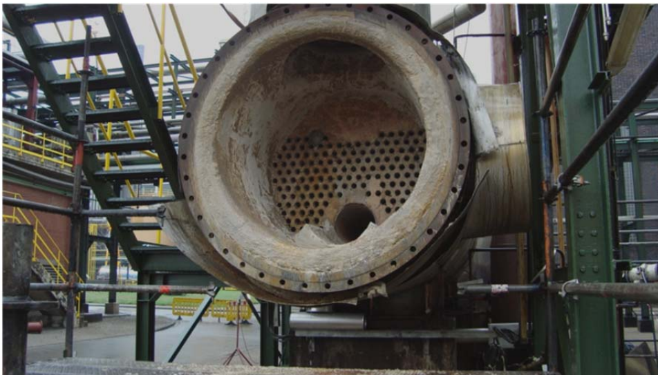
Figure 11. Repaired lining of the waste heat boiler.
