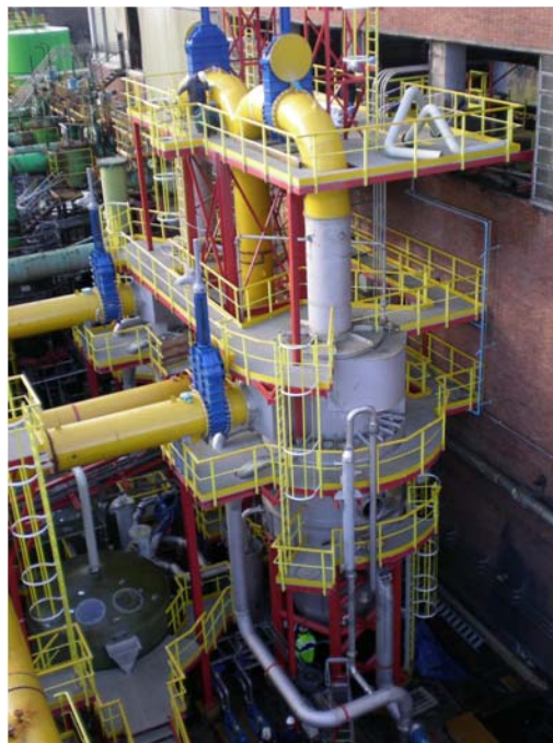
Figure 6. Ammonium sulphate saturator (spray type).
