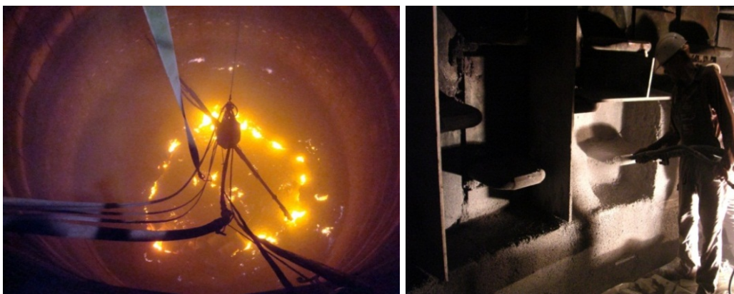
Figure 3: Hot robotic Jetcasting (left) and cold manual Jetcasting from working platform (right).
