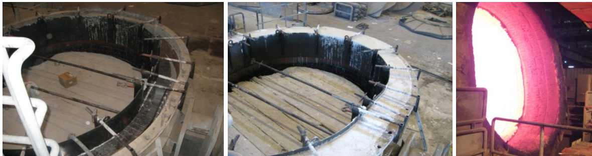
Figure 6: Steel ladle before and after casting the edge covering with Nanobond (top) and after 16 (lower left) and after 65 batches (lower right).
