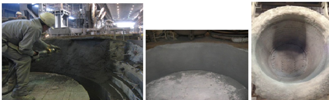
Figure 5: Nanobond Jetcasting of the edge covering of iron ladles.
