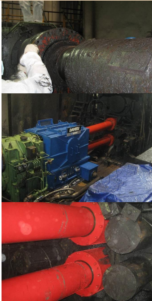
Figure 15. Before and after gear spindle replacement on HSM F7 finishing stand.
