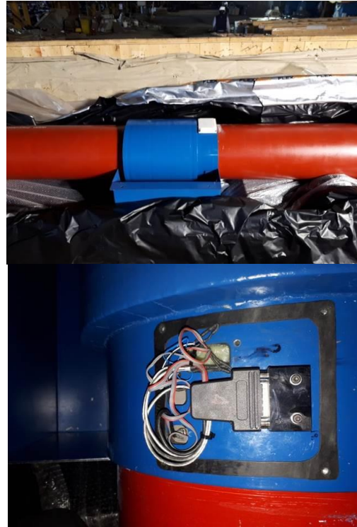
Figure 16. Torque Monitoring Off-line Set-up
