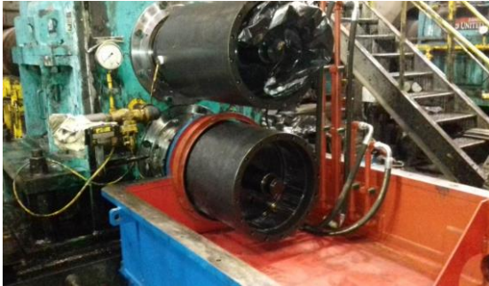
Figure 18. Bottom Frame and Piping
