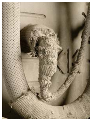
Figure 1: Example of a heat protected sensor mount at the furnace panel.
