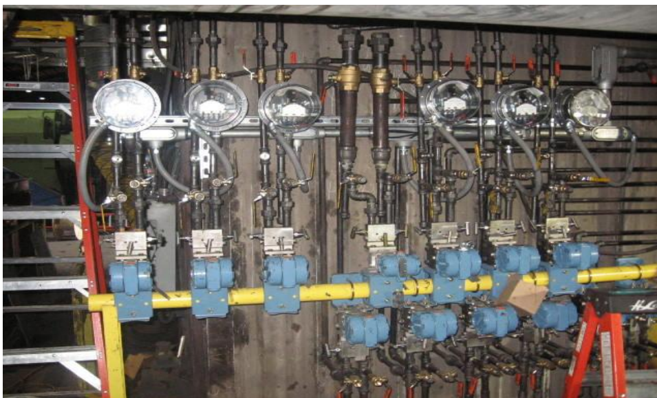
Figure 21: Transmitter Mounting
