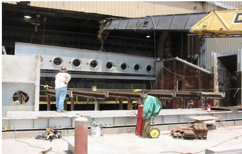
Figure 7: One-Piece Burner Wall Section Being Installed
