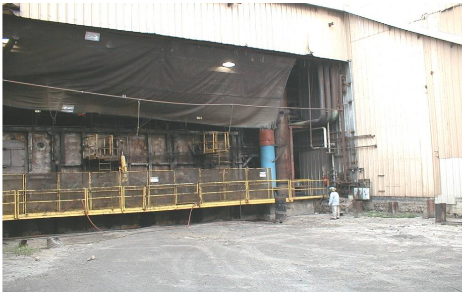
Figure 3: Furnace Charge Area – Limited Construction Access
