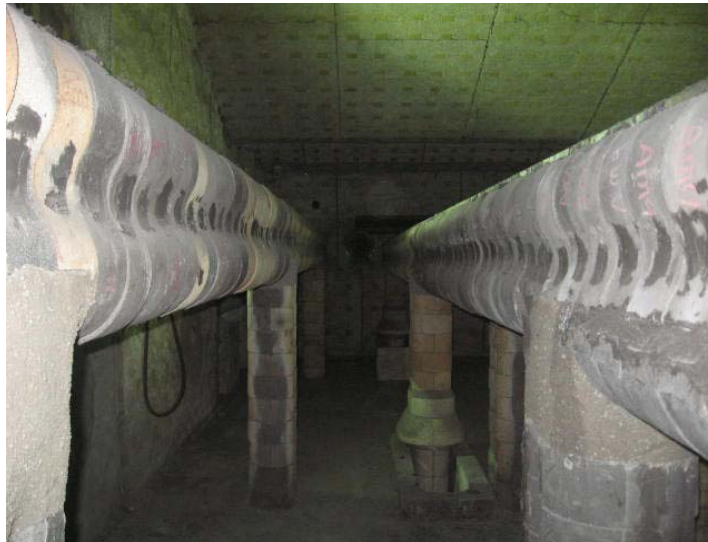
Figure 15: New Refractories Installed
