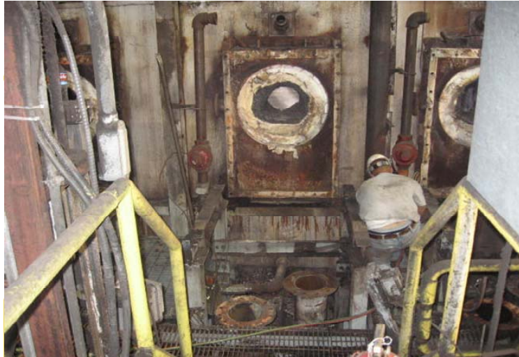
Figure 11: Existing Regenerative Burner Being Removed.
