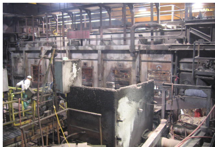
Figure 16: Old Steel Work and Piping Being Removed
