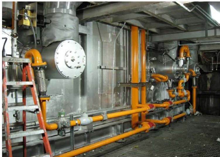
Figure 12: New Burners Installed
