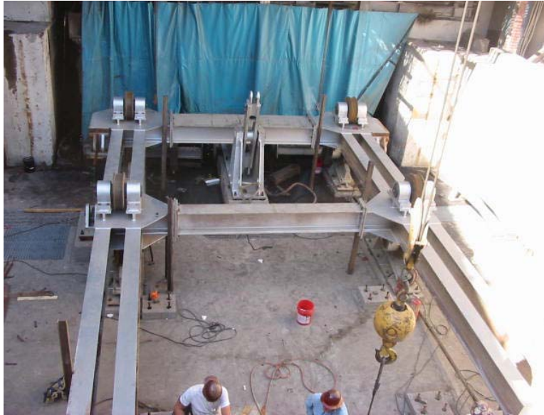
Figure 6: Furnace Charge End Extension – Walking Beam Mechanism Lift Frame
