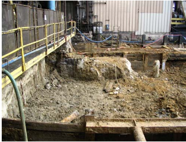
Figure 4: Furnace Charge End Excavation
