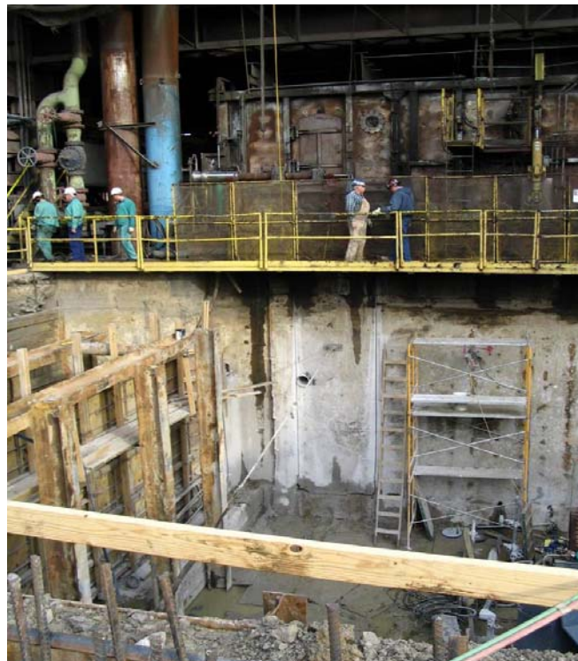
Figure 5: Furnace Charge End Excavation – Foundation Forms
