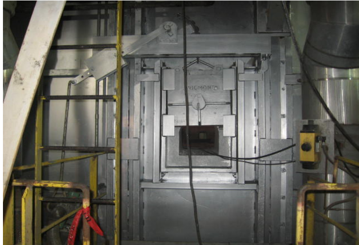
Figure 17: New Steel Work Installed
