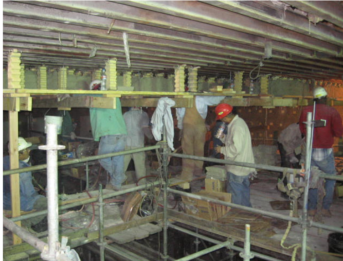
Figure 14: New Refractories Being Installed
