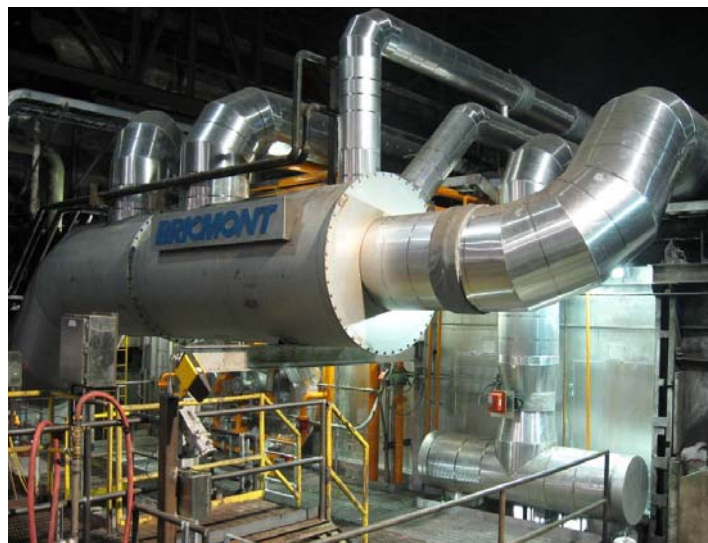
Figure 18: New Piping Installed
