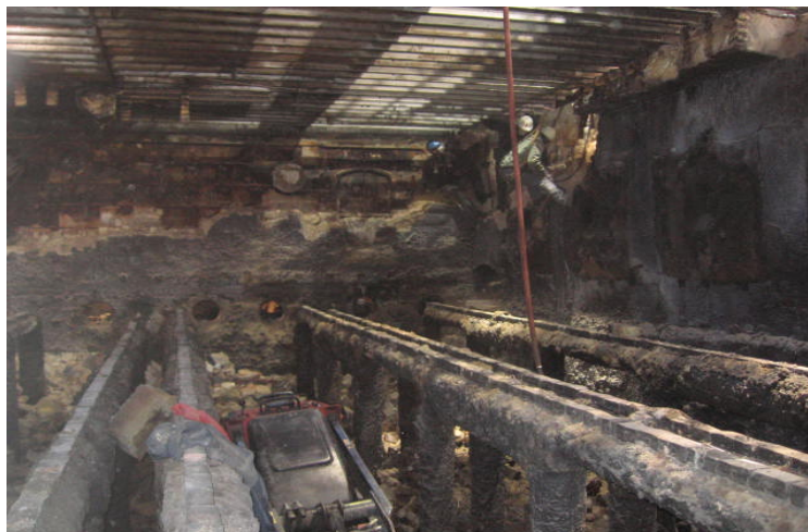
Figure 13: Old Refractories Removed
