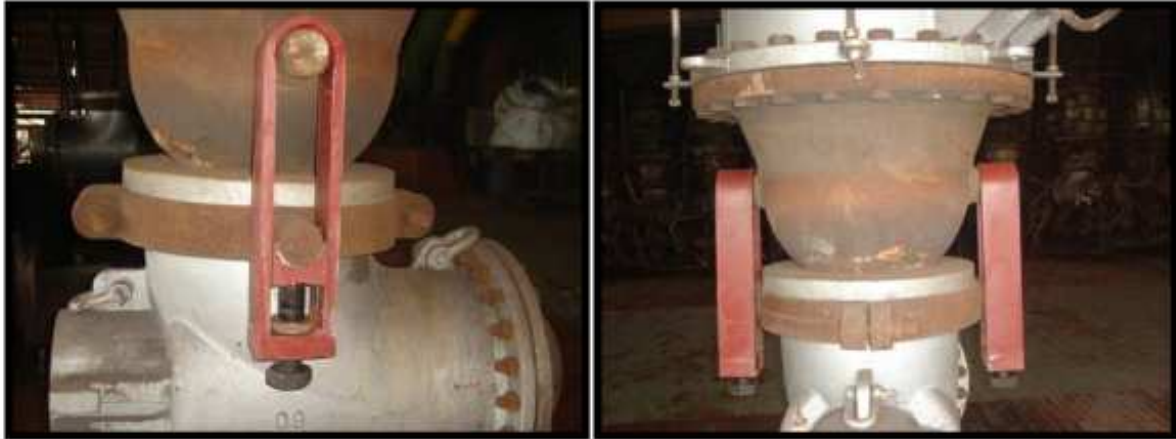
Figure 3 – New Shackle plate assembly.
