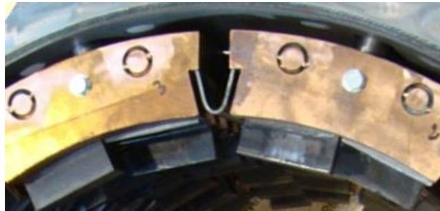
Figure 2.6 Curved stave with in-between blades during erection
