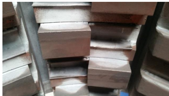
Figure 3.3 Bosh/belly stave design with blades - stone box effect
