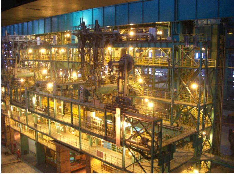
Figure 8. ZHF two180t RH start up (December 2009) plant overview.
