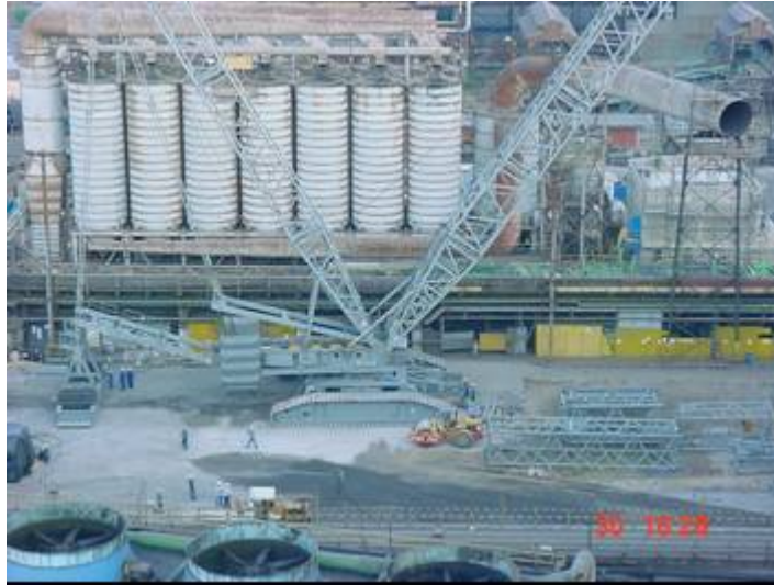
Figure 2. Crane with 240 tonnes capacity.
