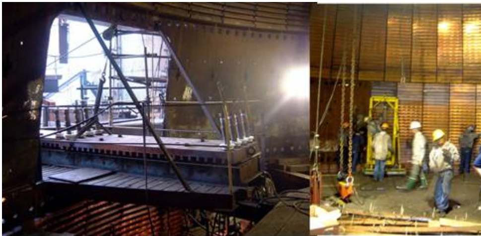
Figure 3. Installation methods for staves.
