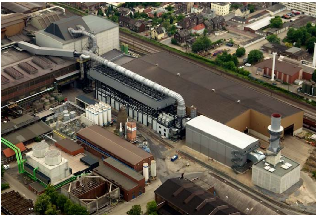
Fig.2: Dedusting plant for Peiner Träger with piping and canopy suction point.
