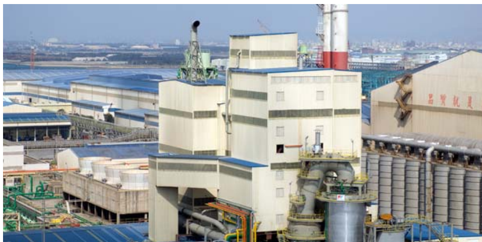
Fig. 16: Primus ® plant at Dragon Steel.
