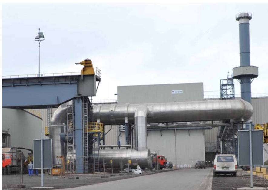
Fig. 6: Heat transformer (front, middle-left) and the bag filter including chimney in the back of the picture, at the Dillinger Hütte, Dillingen Germany.
