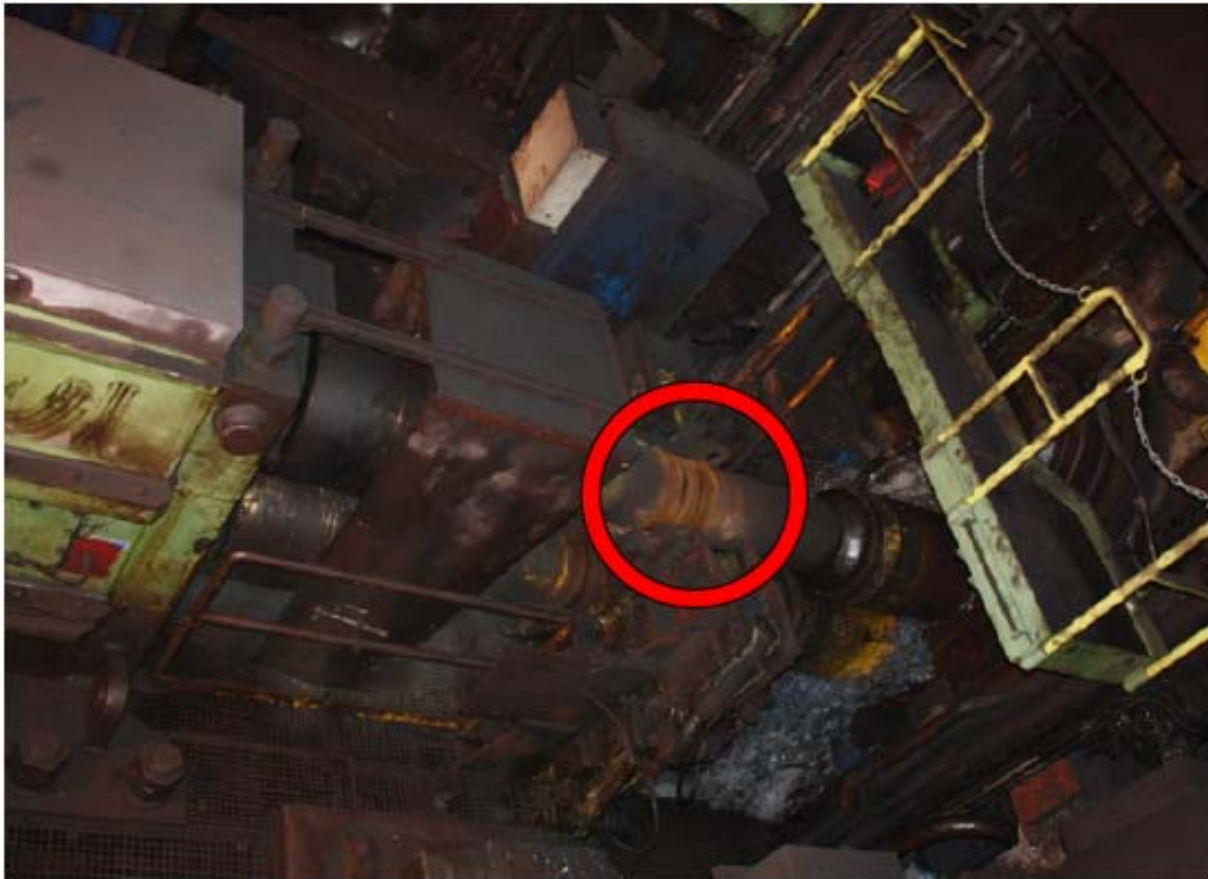
Figure 7: Sensor location at the drive spindles at mill stand 4
