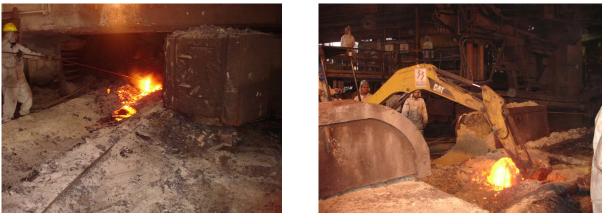
Figure 9 – Main Iron trough filled with sand and the bobcat machine working
