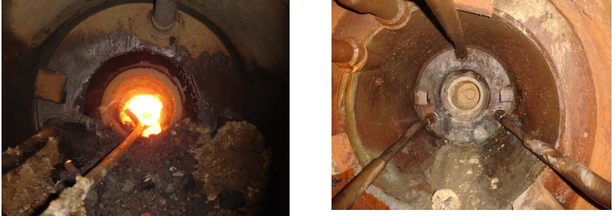
Figure 8 – Tuyere cleaning and preparation
