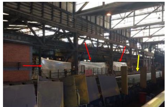
Figure 1 Curtains installed in the cooling bed.
