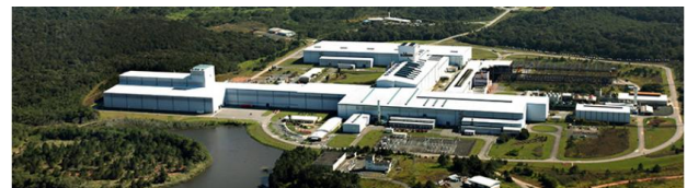
Figure 2.1 ArcelorMittal Vega site
