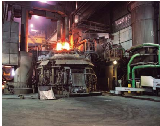
Figure 1 - EAF general view
