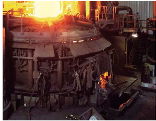
Figure 3 - EAF with side wall injectors
