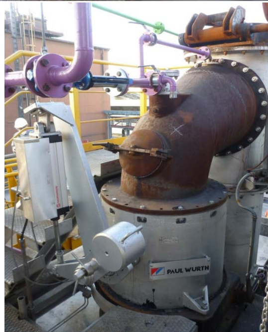
Figure 6. Installation on the New Battery.
