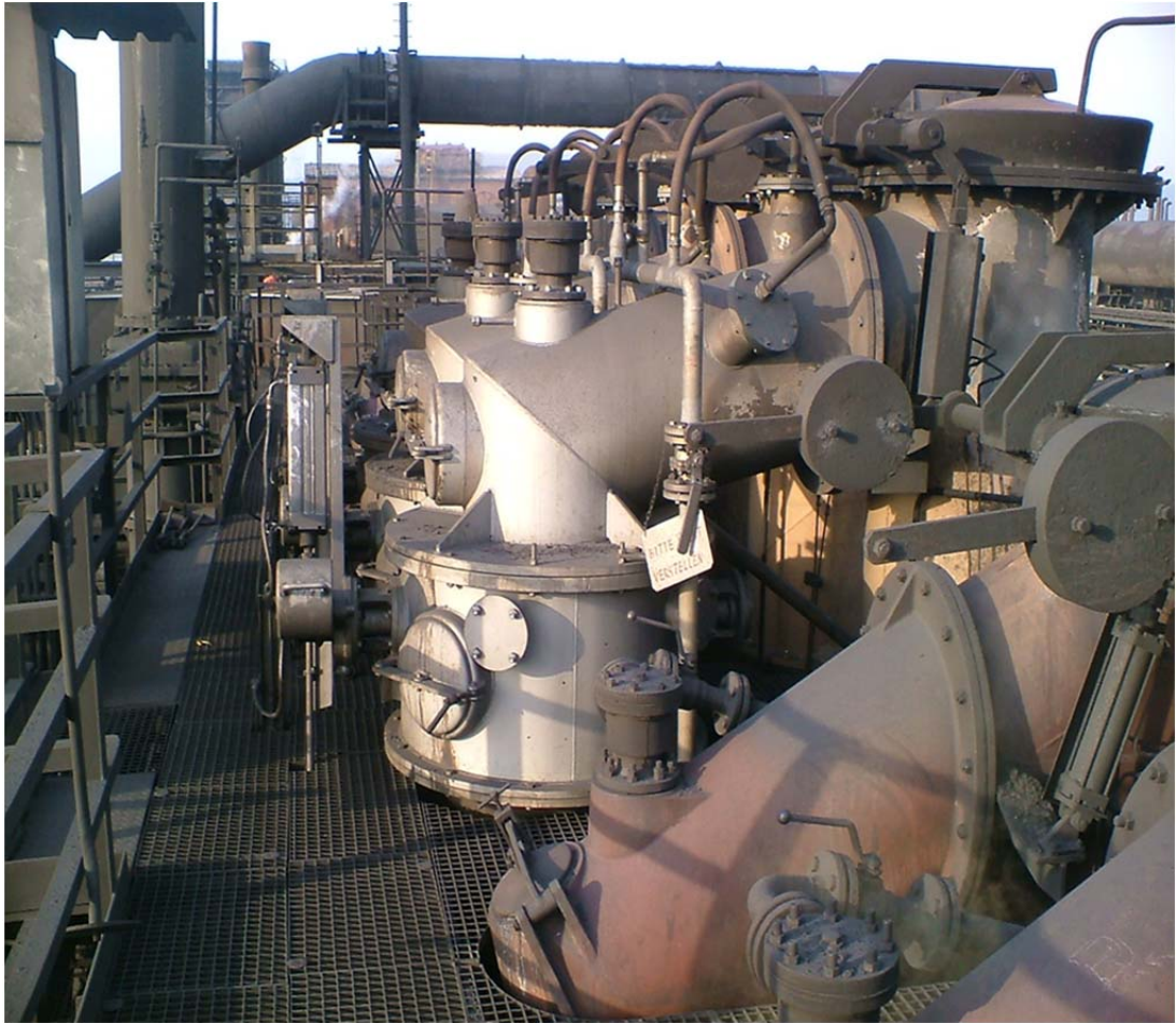
Figure 4. Sopreco ® Valve Installation for Trials.
