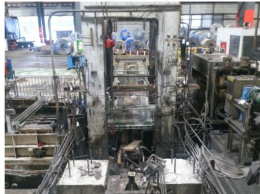
Figure 10a : Skin pass mill completely dismantled
