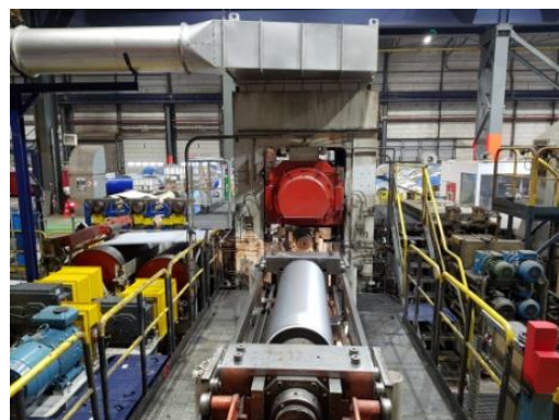
Figure 10b : Same view after revamping
