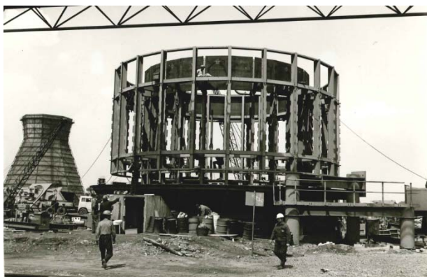
Figure 8: Erection of a shaft cooler at Hüttenwerke Krupp Mannesmann 1971
