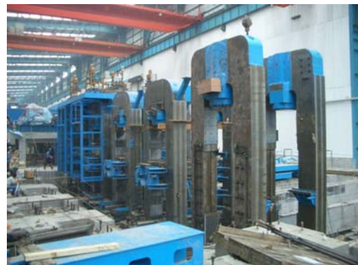
Fig.8 - Erection of stands
