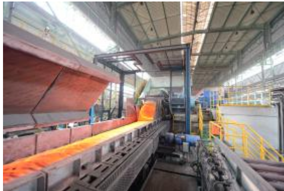
Figure 7. The latest generation LLH in operation at Angang Anshan I&S – P.R. Of China.
