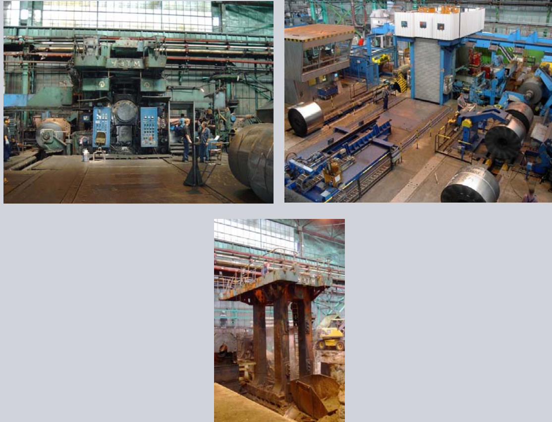
Figure 11: Skin Pass Mill in Dunaújváros, Original, dismantled and modernized mill
