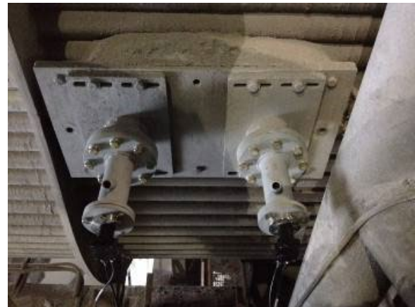
Figure 9. Installation of OVM
