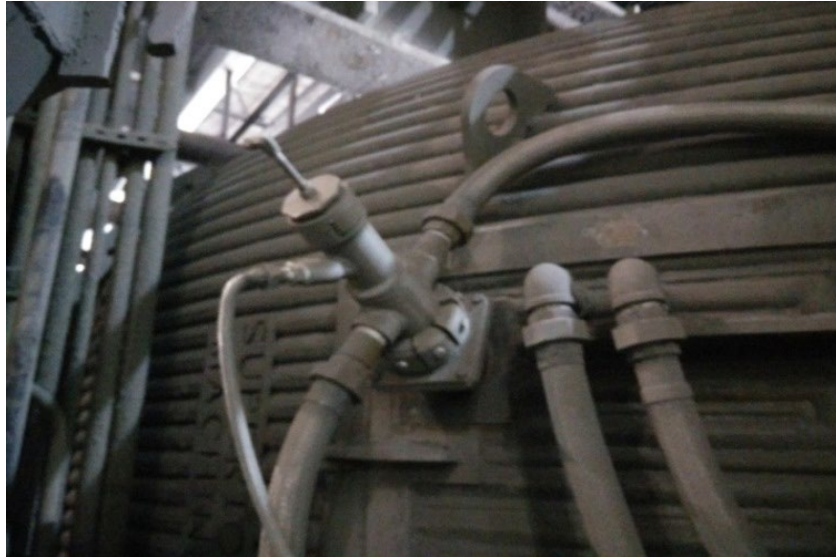
Figure 1. Probe Installation in a water-cooled panel
