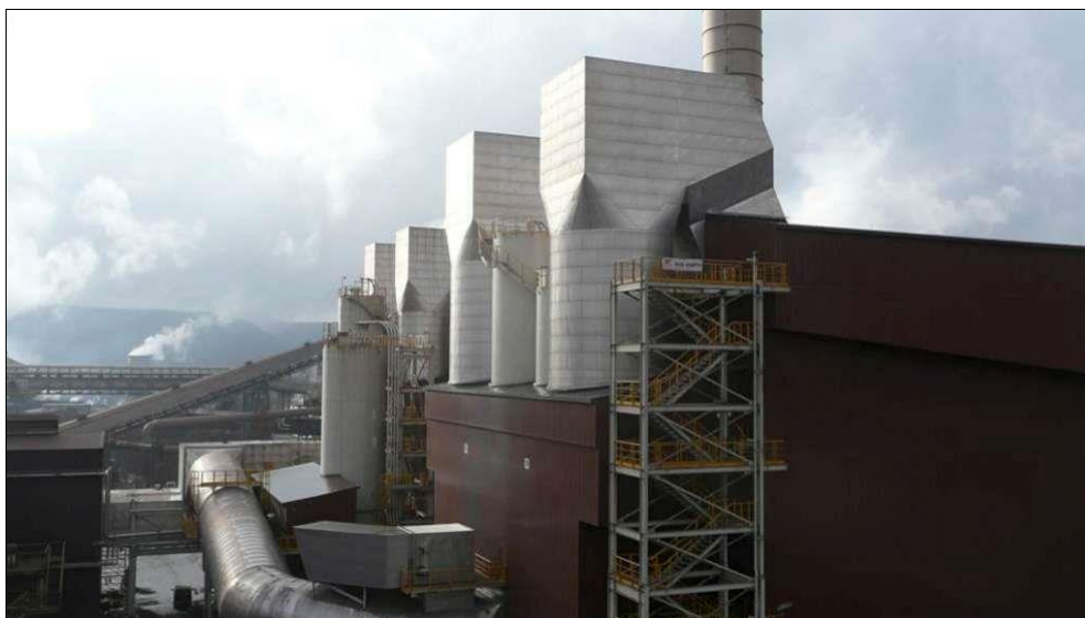
Figure 12: Plant view of the two Rogesa, EFA™ plants.
