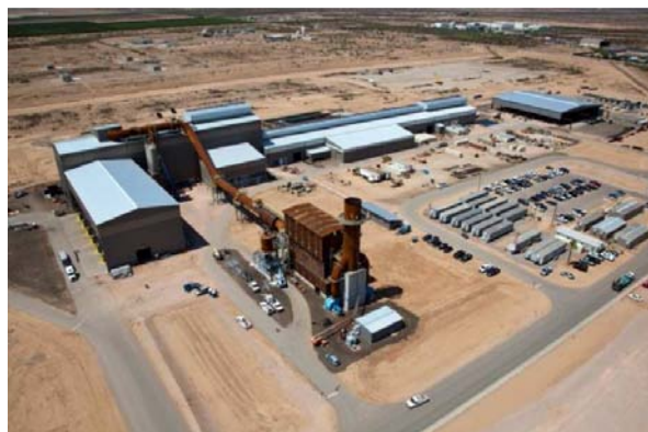
Figure 19. Site prior to commissioning.
