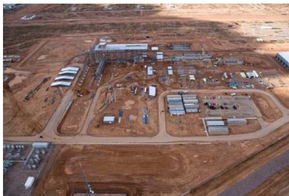
Figure 18. Site midpoint thru construction.
