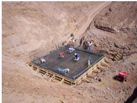
Figure 17. First concrete pour, late 2008.
