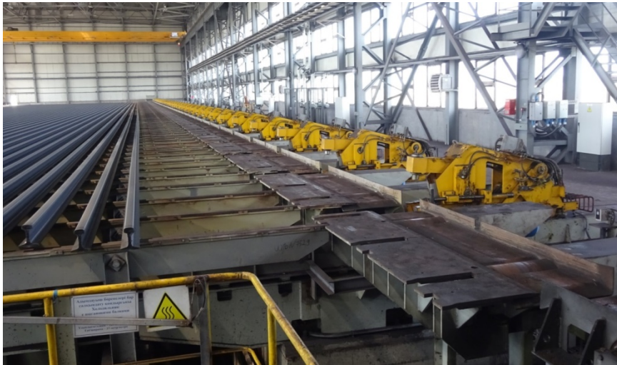
Figure 06. Cooling bed with pre-cambering
