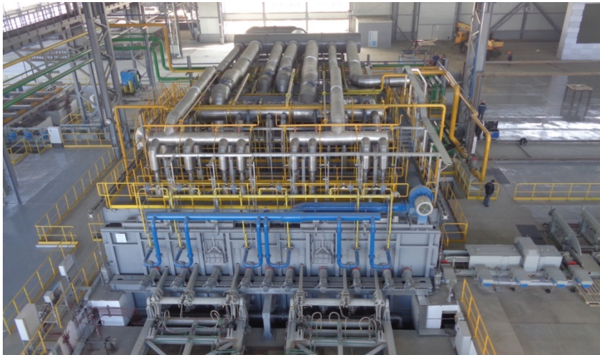
Figure 02. Bloom re-heating furnace
