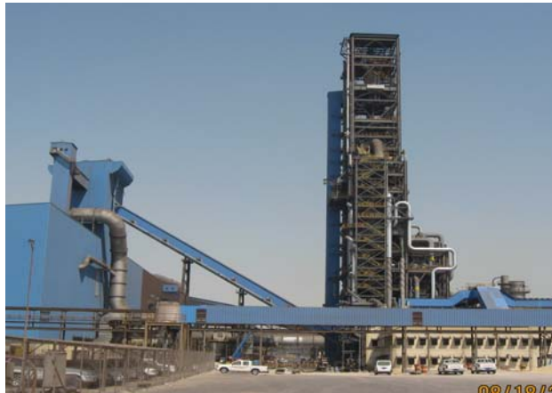
Figure 9: Picture of DRI and Steel Making plant
