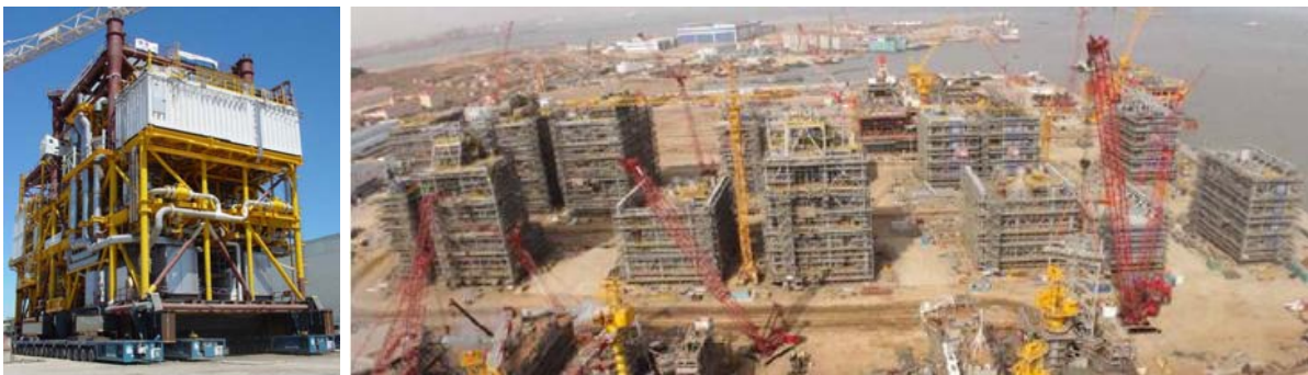
Figure 1. (a) Module being transported by SPMT; (b) Modules fabrication yard. (2)
