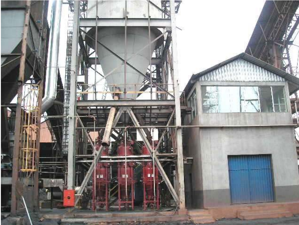
Appendix 07: view of the PCI installation (process silo + control room)
